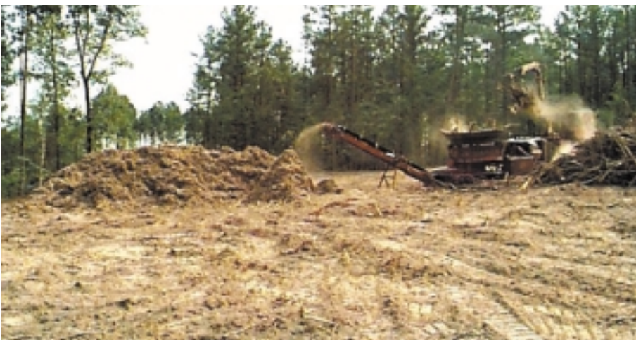
Debris grinding with tub grinder
