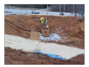
Steeper slopes were covered with woven straw mats to slow erosion and then seeded with a grass mixture. Natural drainage courses on steeper slopes were covered with cobbles to slow water flow across the surface.
