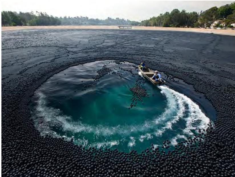
**Figure 3.11:** Dark polyethylene (PE) spheres at the air-water interface to reduce the level of bromate in Ivanhoe clean water reservoir. Image taken from [Ivanhoe, 2011].
