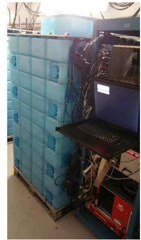
Array with water shielding at ORNL.
