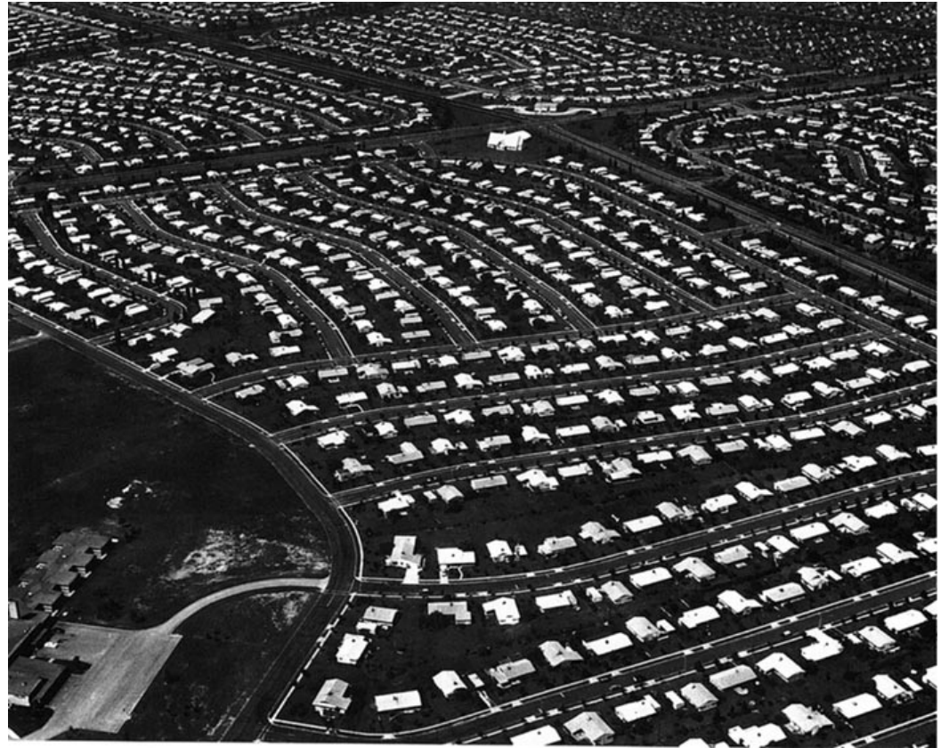
Aerial view of Levittown, Pennsylvania circa 1959. https://en.wikipedia.org/wiki/Levittown .
