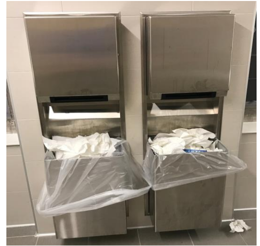
Craven VO bathroom (renovated 2019)
