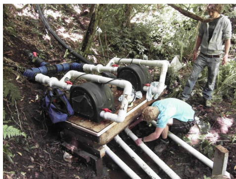
Installed PowerSpout system
