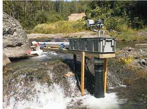
Installed turbine with the sluiceway
